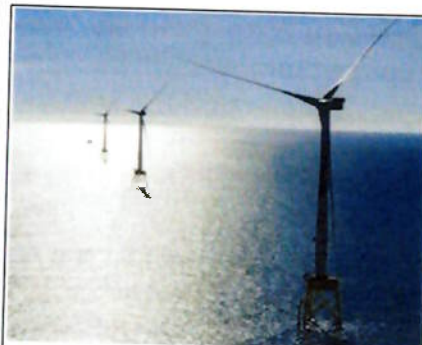
Image 7 Typical WTG on a Jacket foundation (Source: CIP)
